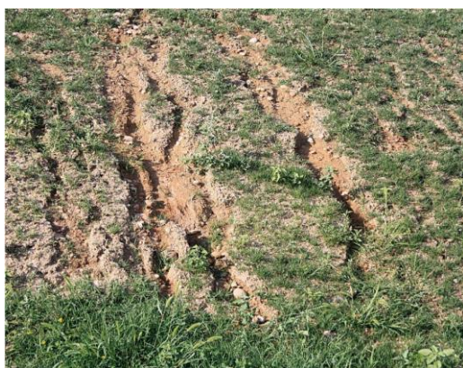
FIG. 3 Erosion on areas next to traffic routes. A vegetation cover serves as erosion protection on many “Eh da” areas close to transport routes, which is non-existent in this example.
