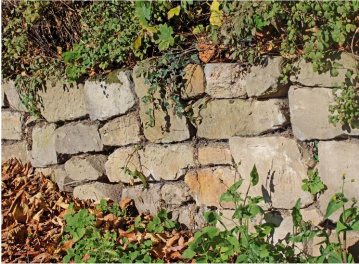
FIG. 10 Stones form a structure in a landscape. Clearance cairns and rock walls are important structural elements in a landscape used by many different animals. Locally sourced rocks are preferable when laying out these areas. Structures such as gabions (mesh wire cages), which have become immensely popular in the last years, fail to provide suitable habitats for animals due to their shallow depths.
